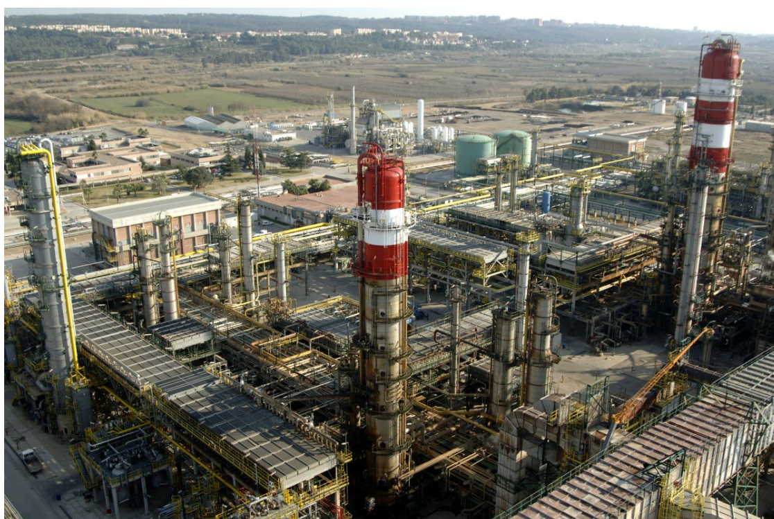
El Complex Industrial de Repsol a Tarragona | Repsol
